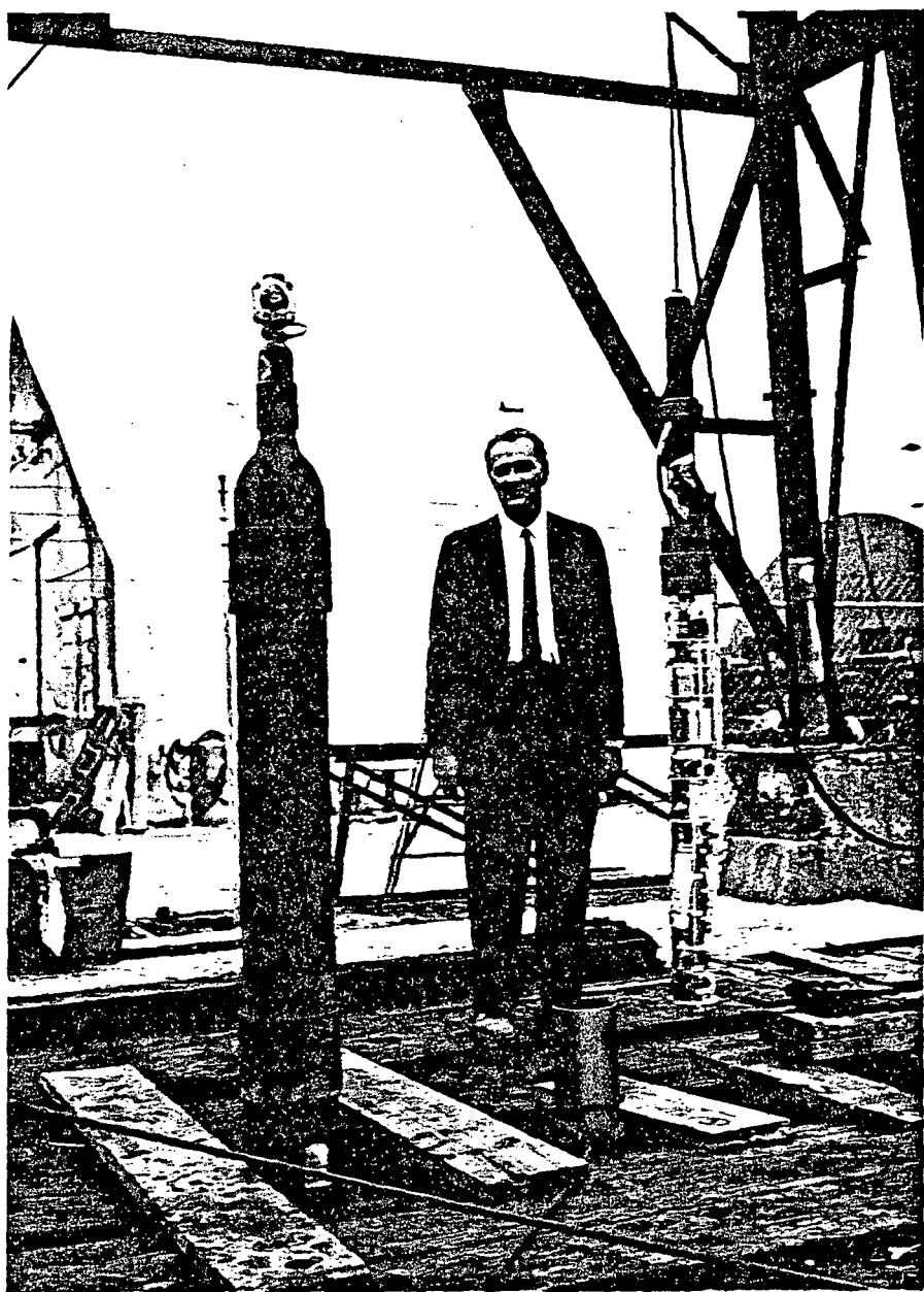
Figure 2. Dr. Lucien LaCoste standing beside the LaCoste & Romberg Company's borehole gravity meter No. 1 which is hanging outside of its pressure housing, Santa Fe Springs oil field, California, March 24, 1966, less than two weeks before the first fully successful well test.
