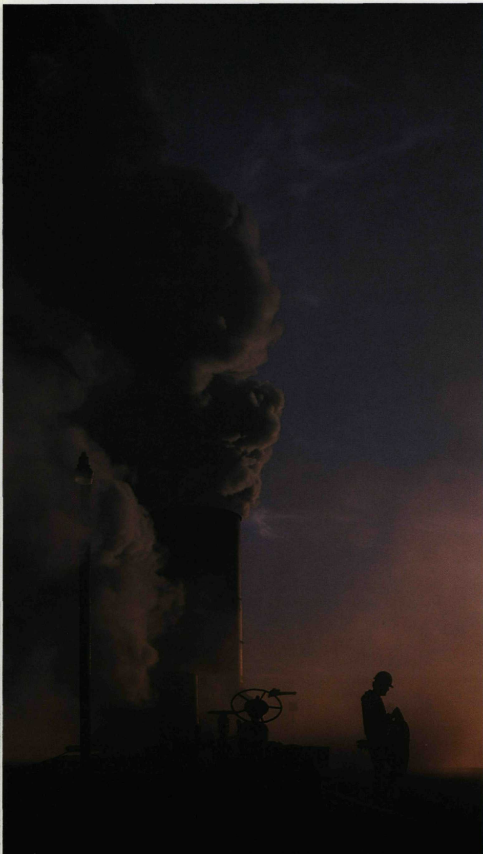
The drift of Baja California away from the main mass of Mexico has created a geological hot spot beneath the Salton Sea, which scientists think may be an enormous untapped power resource
