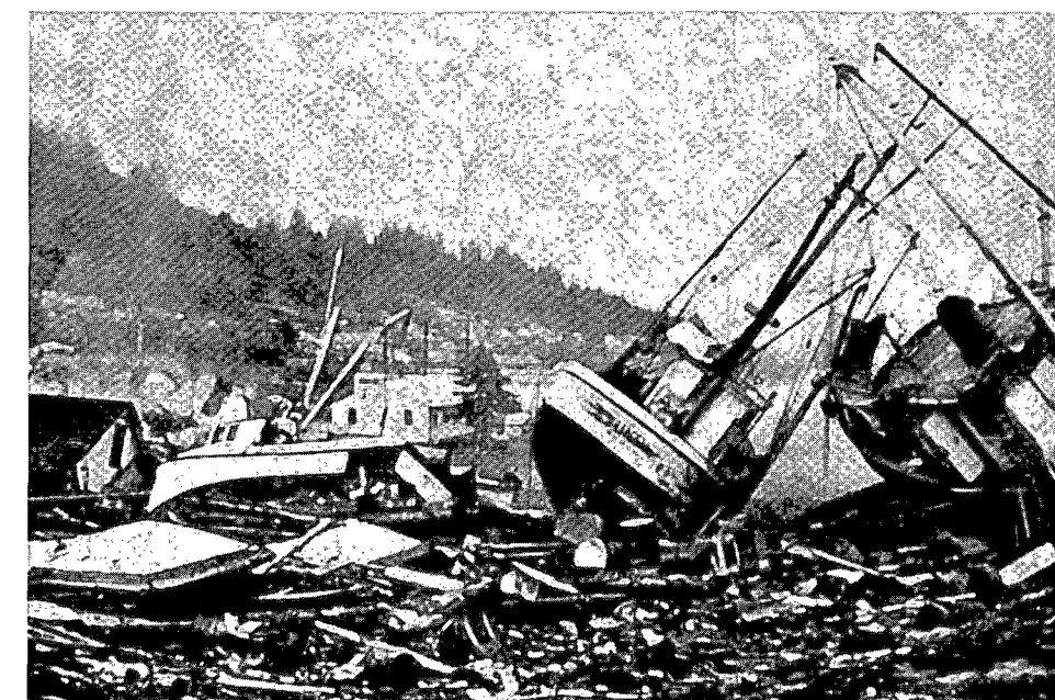
Tsunami Damage at Seward, Alaska, Port Facilities (March 1964).
