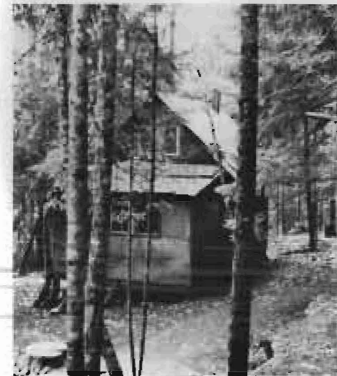
ONE of two buildings removed by BLM near Galice, Oregon.
