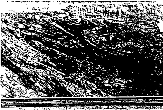
FIGURE 9. Top: successful pre-splitting with the predominant discontinuity set orientated perpendicular to the face.
