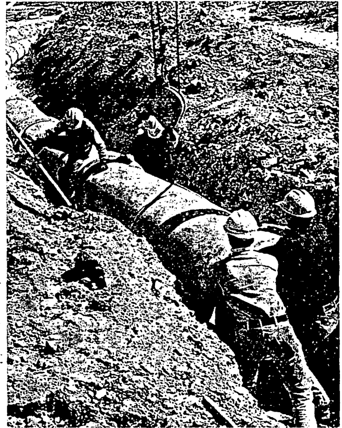
Transite asbestos-cement pipe (36-in.) carries pregnant solution from the dumps to the precipitating plant. Workmen lay a section with Ring-tite couplings which permit deflection.
