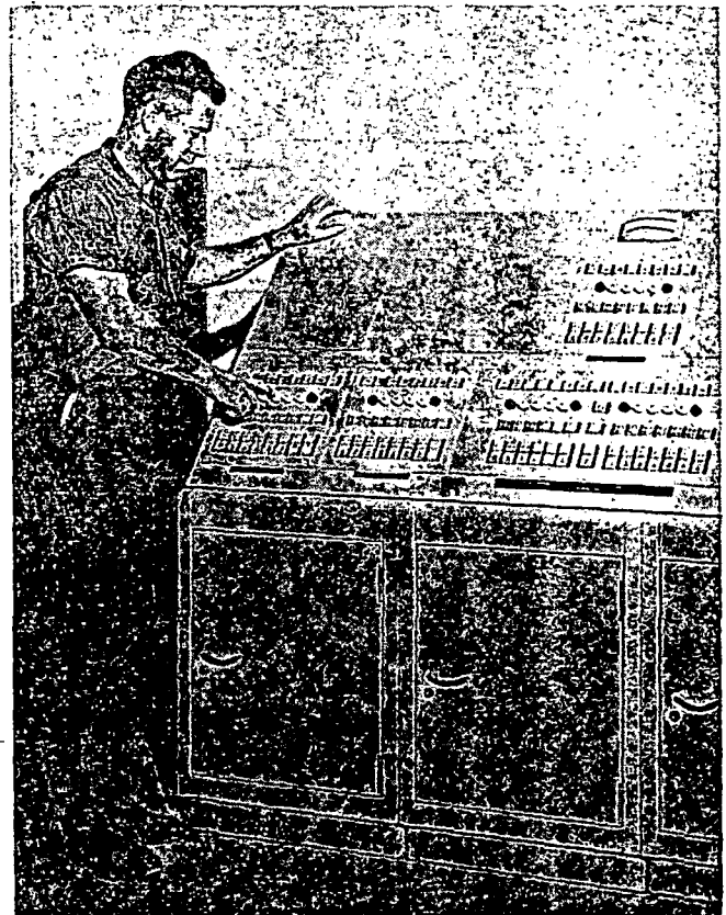
The control center for the leach-solution distribution in the precipitating plant operations building.
