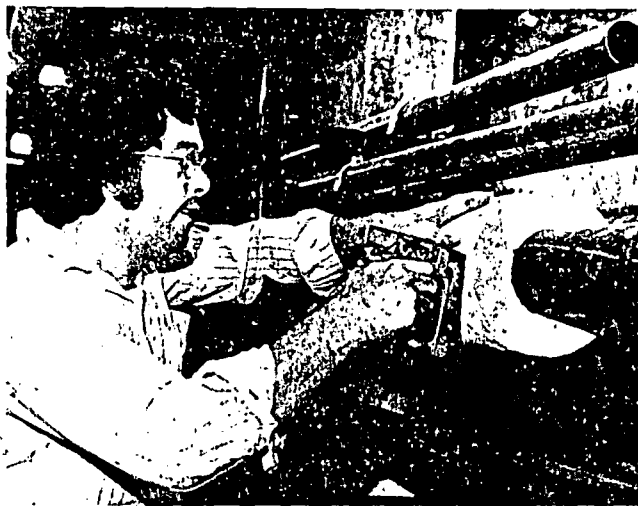
First step in installing glass fiber pipe insulation is to slip it over the pipe (top). The closure flap is stapled down after the insulation is in place (courtesy of TIMA).
