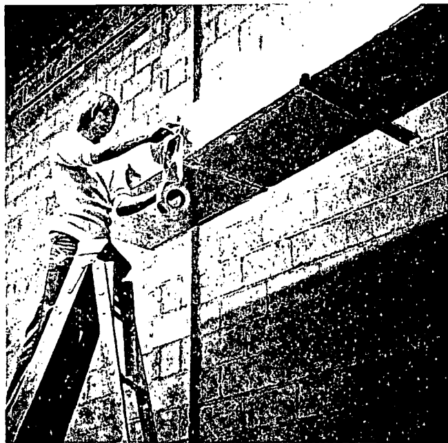
Lightweight glass fiber duct sections are lifted into place and connected to other sections (courtesy of TIMA).
