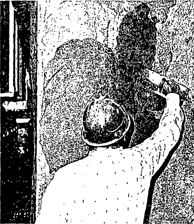
Insulating cement is troweled into place. In this instance, the insulation is being applied to a breaching in a utility shaft (courtesy of TIMA).
