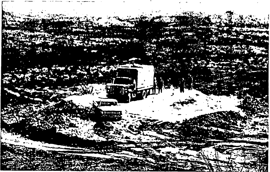
FIGURE 3.- Blasthole loading.
