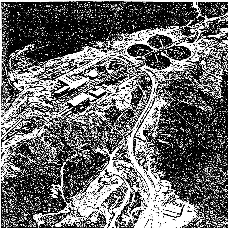
Cyanidation plant at Pueblo Viejo mine in Dominican Republic. Facility was designed to treat 8000 tpd of gold and silver bearing oxide ores
