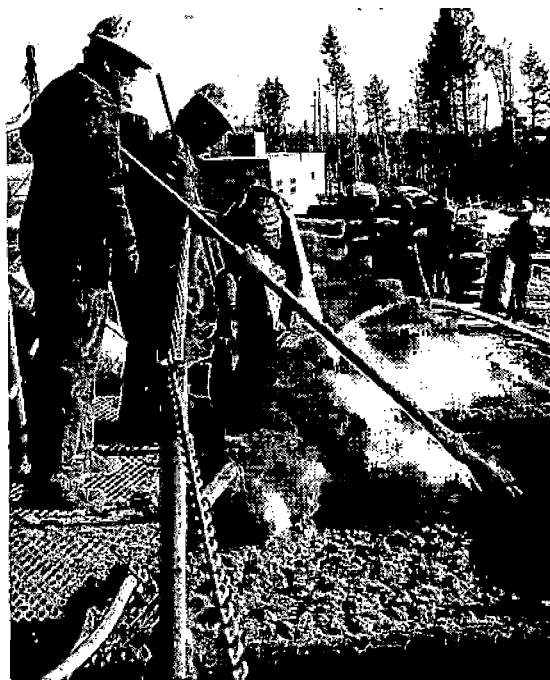
Fig. 9. Mixing drilling mud in the drilling rig mud tanks. Mud testing trailer is seen in the background.
