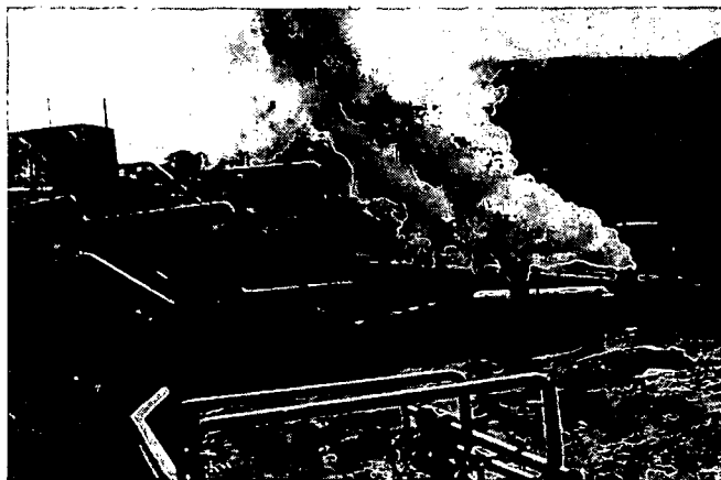
During temporary plant shutdown, steam is vented through large mufflers to keep gathering system and wells at proper temperature. Intermittent operation is avoided as wells are sensitive to shut in and start up. Occasional system shutdown gives opportunities for reservoir pressure build-up tests.
