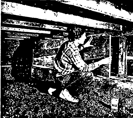
Foundation cripple walls should be sheathed with plywood to reduce chance of collapse in a quake. Where sill is a 2 by 6, add blocking as shown to create flush surface for nailing. If sill is a 2 by 4, you can nail the plywood directly to it. To prevent condensation, cut ventilation holes (not necessary if insulation is added)
