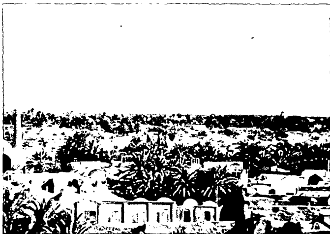
A. TABAS BEFORE ITS DESTRUCTION. THE BUILDINGS CONSISTED OF MASSIVE ADOBE WALLS AND DOMED ROOFS, WITH DATE PALMS IN THE COURTYARDS.
