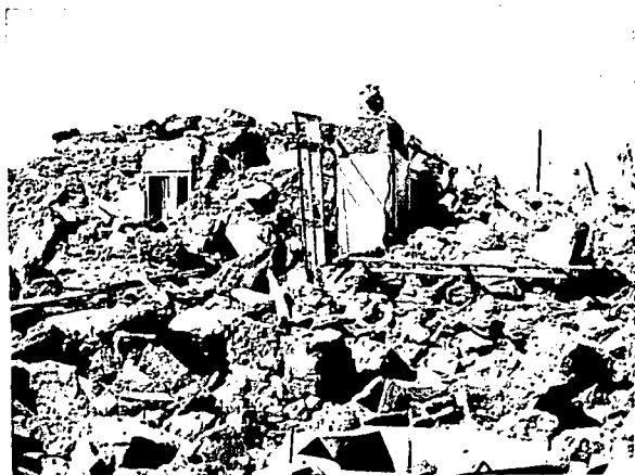
C. THE COLLAPSE OF ADOBE BUILDINGS PRODUCED HIGHLY FRAGMENTED MOUNDS OF RUBBLE.
