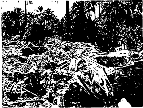
D. PILES OF RUBBLE AND DEBRIS MARK THE SITE OF BUILDINGS.
