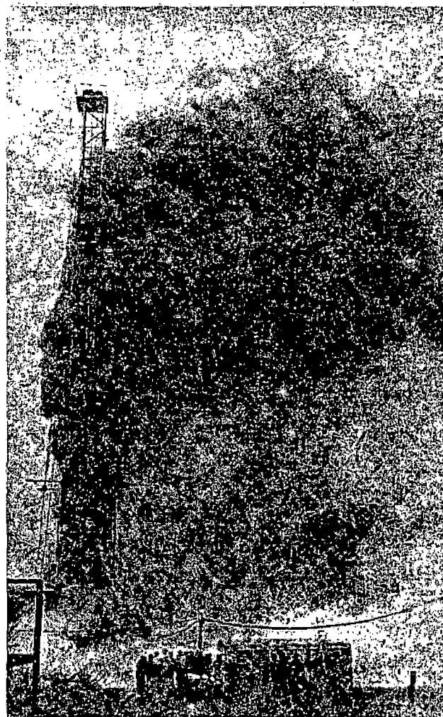
Fig. 12. — View of the Alfina 1 well, 36 hours after explosion. The steam-gas jet is carrying a remarkable amount of dust and chips.
