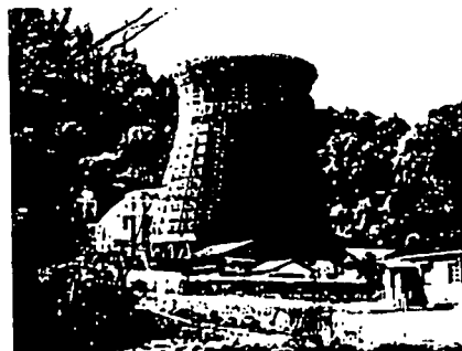
Cooling Tower of Matsukawa
