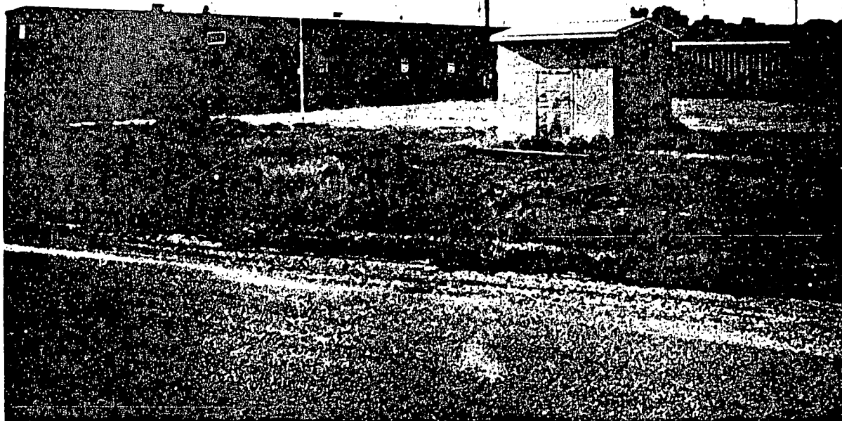
Figure 2. Photograph of the municipal well at Midland, S. D. The small building in the foreground houses the Midland city well. Hot water from this well heats the gymnasium in left background and the classroom building in right background.
