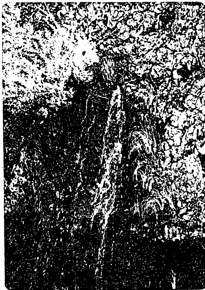
FIGURE 26. Road cut and emerging water streams from thin diktytaxitic flows in the lower High Cascade volcanics, in road cut at Trail Bridge Reservoir, North Fork of the McKenzie River.
