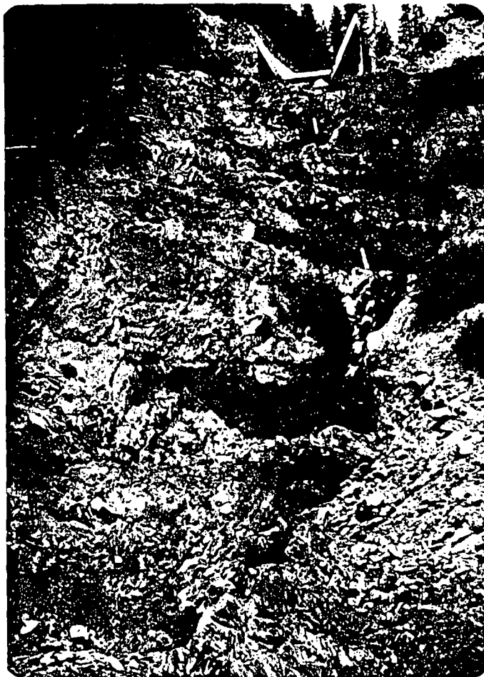
FIGURE 6. Spillway at Smith River Reservoir, showing numerous thin lava flows interbedded with volcanic tuffs and breccias.
