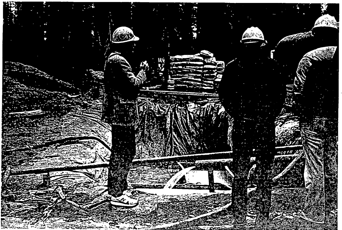
BLM AND NPS INSPECTION OF SUMPS AND CORE DRILLING WATER
