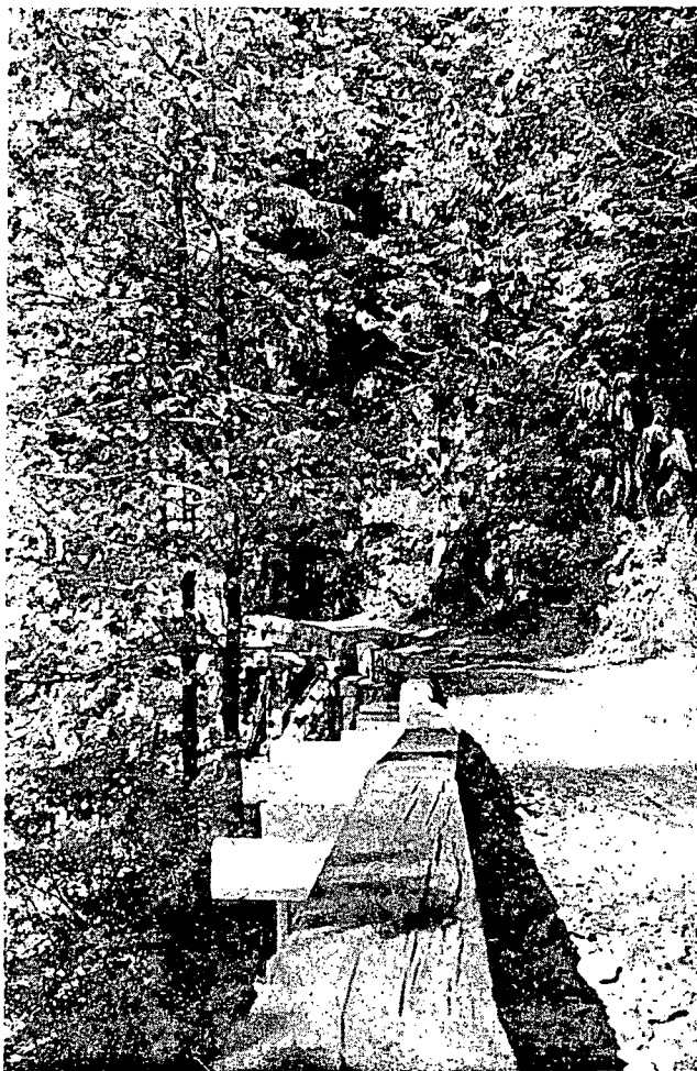
Stop 2. Half bridge, so called because the road is supported on one side by timbers and the other by the side of the valley, was required where the highly resistant rock of a large intrusion was encountered by the early miners in the North Santiam mining area.
