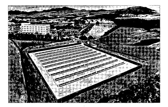
A photovoltaic system, capable of producing up to 40 kilowatts of electricity, is being installed at the G.N. Wilcox Memorial Hospital on Kauai. Funded by the U.S. Department of Energy and the State of Hawaii, the project has the participation of HNEI, Kauai County, Kauai Electric Company, Wilcox Hospital, and Acurex Corporation, the system designers.
