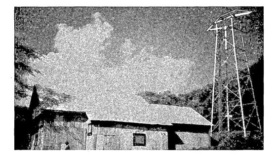
Hydroelectric plants in Hawaii are run-of-river plants; they use available stream flows without dams. Run-of-river plants without storage use the water directly as it comes through the stream to turn a turbine and generator to produce electricity. Most run-of-river plants in Hawaii are capable of maintaining a base electrical load throughout the year because there is always at least a minimum flow of water.
