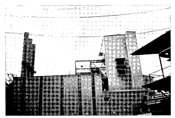
Bagasse boilers are not new in Hawaii. In fact, sugar plantations rely upon the electricity produced by the bagasse burning to provide most of their electrical needs, selling any excess to the local utility. The new bagasse boiler in Lihue is special because of its emphasis; it was built with the utility as well as the plantation in mind. The new plant has enabled the utility to defer buying a new oil-fired generating plant.
