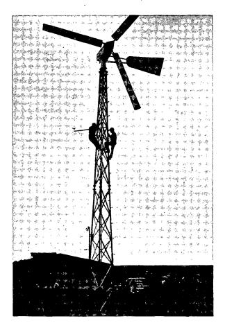
A Millville wind energy conversion system (WECS) has been installed on the Hawaiian Homestead Commission land of Bucky Davis on Molokai. The WECS, with an estimated capacity of 10 kilowatts, has been producing an average of 23.91 kilowatt hours a day, or just under 1 kilowatt per hour. This is slightly more than the family uses.
