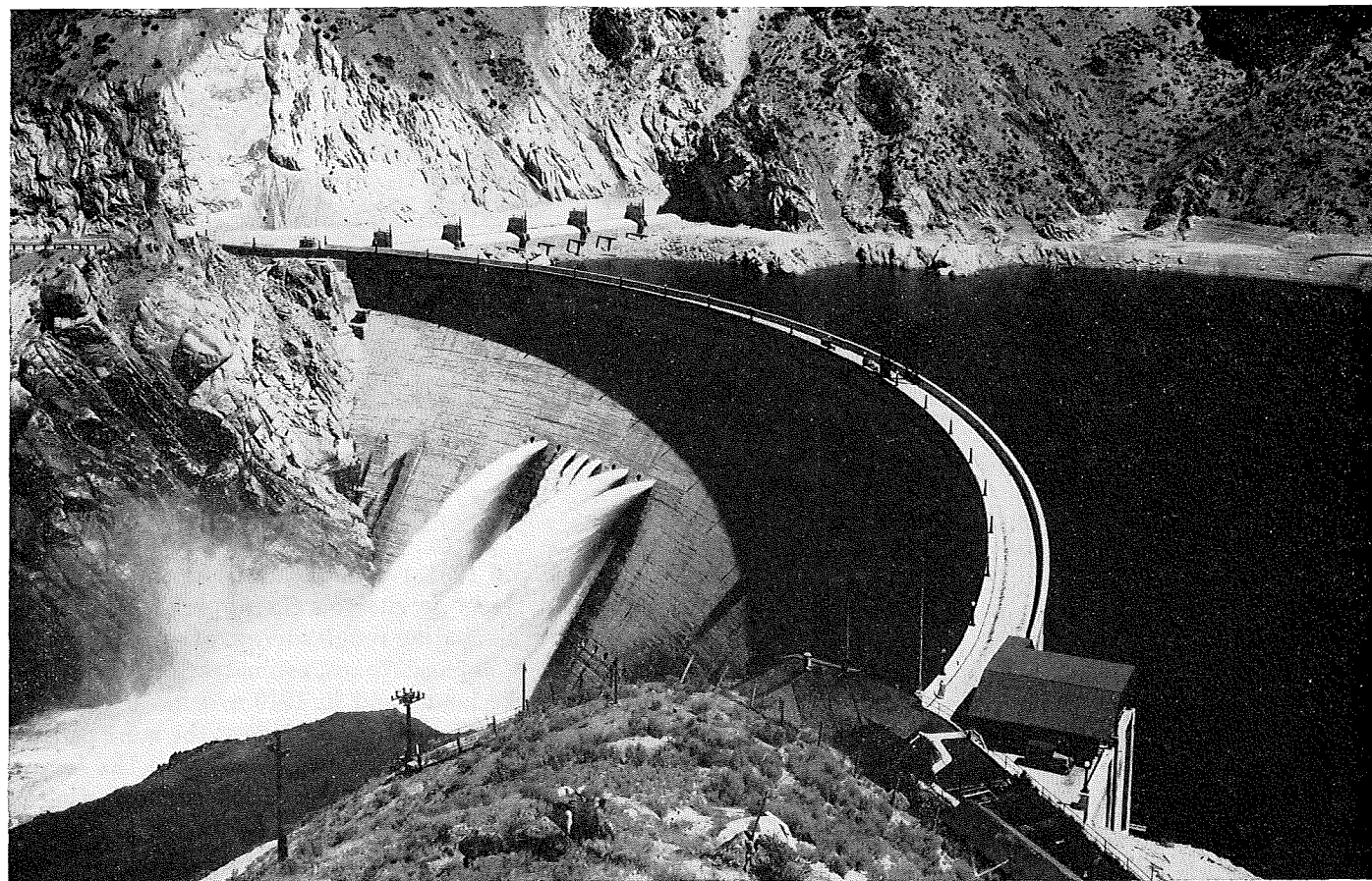
With Arrowrock Reservoir at a low stage, irrigation water for the Boise project pours from the upper tier of outlets.
