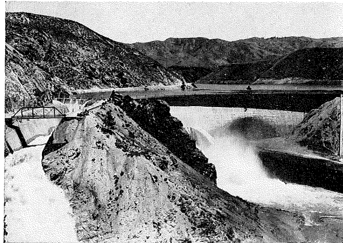
Arrowrock spillway discharges beneath the bridge on the left, and the outlet works discharge into the river channel in the center. The chute at the right is the logway, by which saw timber is passed over the dam.
