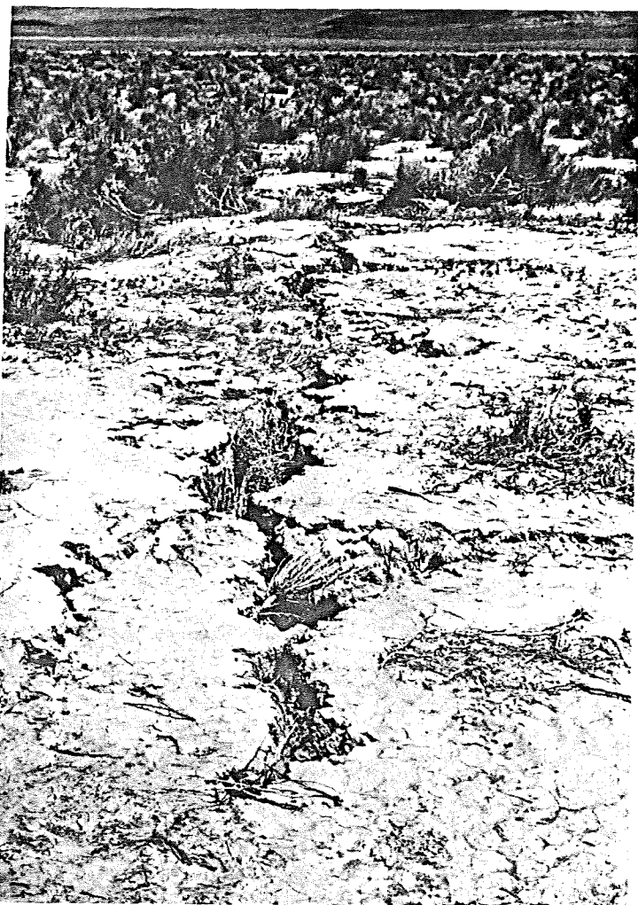
Figure 2.—View north-northeastward along a portion of a 1,200-ft-long (360 m) tectonic rift (surface crack) in central part of Hualapai Flat. Photo taken in summer 1975. (Photo: LTG 24775)
