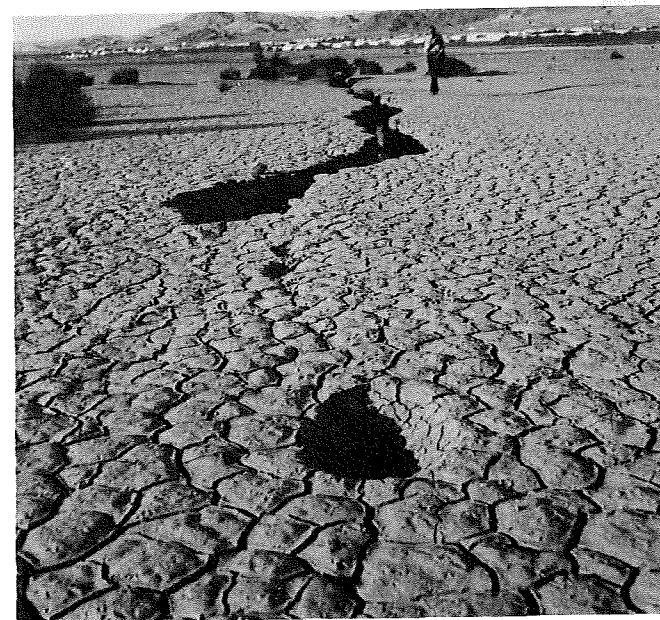
Photo 3. Fissure "healing" in a manner similar to giant desiccation cracks. Looking north toward unnamed northwest trending fault.
