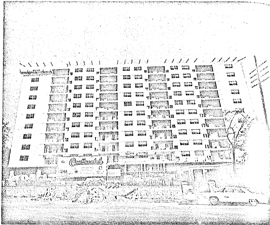
In applications of this type at Continental Apartments, Nashville, Tennessee, each apartment and each commercial area on the ground floor can be individually equipped with heat pumps to provide year-round heating and air conditioning comfort. In this case, each apartment has its own individual comfort system.
