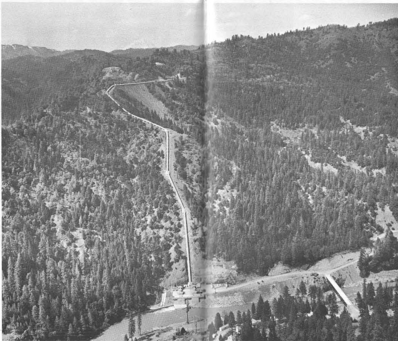
Water reporting for work takes a long fall inside big steel pipes like this penstock above James Black Powerhouse on the Pit River in Shasta County. The waterflow builds up terrific pressure (called head) in descent. Spurting from nozzles at the bottom of the penstock at speeds up to 200 miles per hour, the waterflow strikes the blades or buckets on waterwheels. These in turn spin the energy-making generators. No water is wasted or consumed in generating hydroelectric power.
