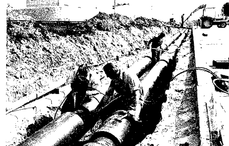
Insulated heating pipe sections prevent heat loss
