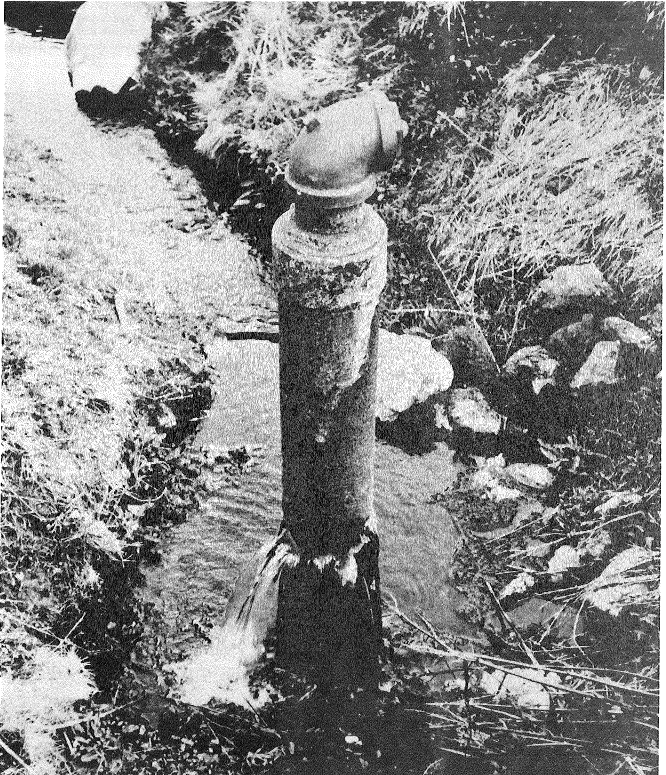
Abandoned well (Sample 1) on the Fort Bidwell Indian Reservation. Water at 45.1°C flows from holes in the corroded steel pipe. Photo taken October 1973.
