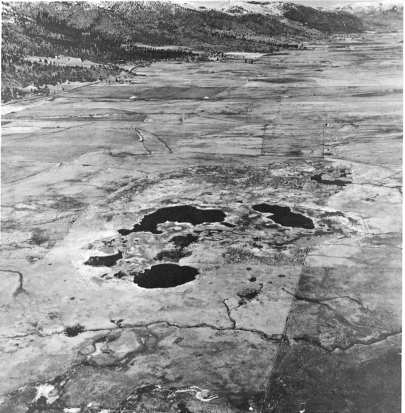
View northward of the Lake City mud eruption area on the west side of Surprise Valley. Lakes in the foreground occupy craters formed during mud and steam eruptions in 1951. Hot springs presently discharge beneath the lakes and in the surrounding marsh. The Warner Range in the background has been uplifted along the Surprise Valley fault. Photo by R. E. Franson, Dec. 1960.
