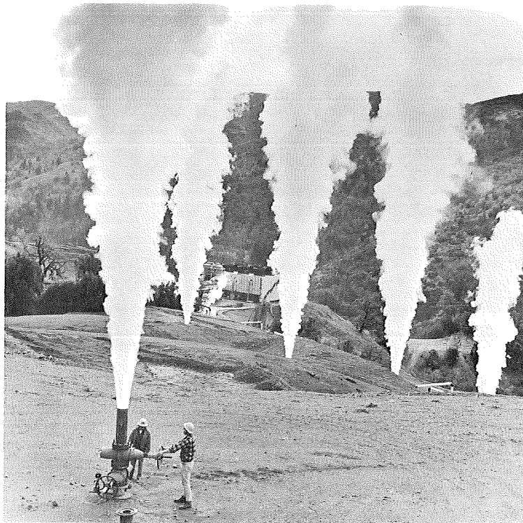
Photo No. 4. Pacific Gas and Electric Company engineers study the pressure and temperature of this geothermal steam well at PG&E's The Geysers Power Plant in Sonoma County, California. Wells to produce steam for the plant have been drilled to a depth of more than a mile and a half. Behind the steam wells can be seen Unit 3.
