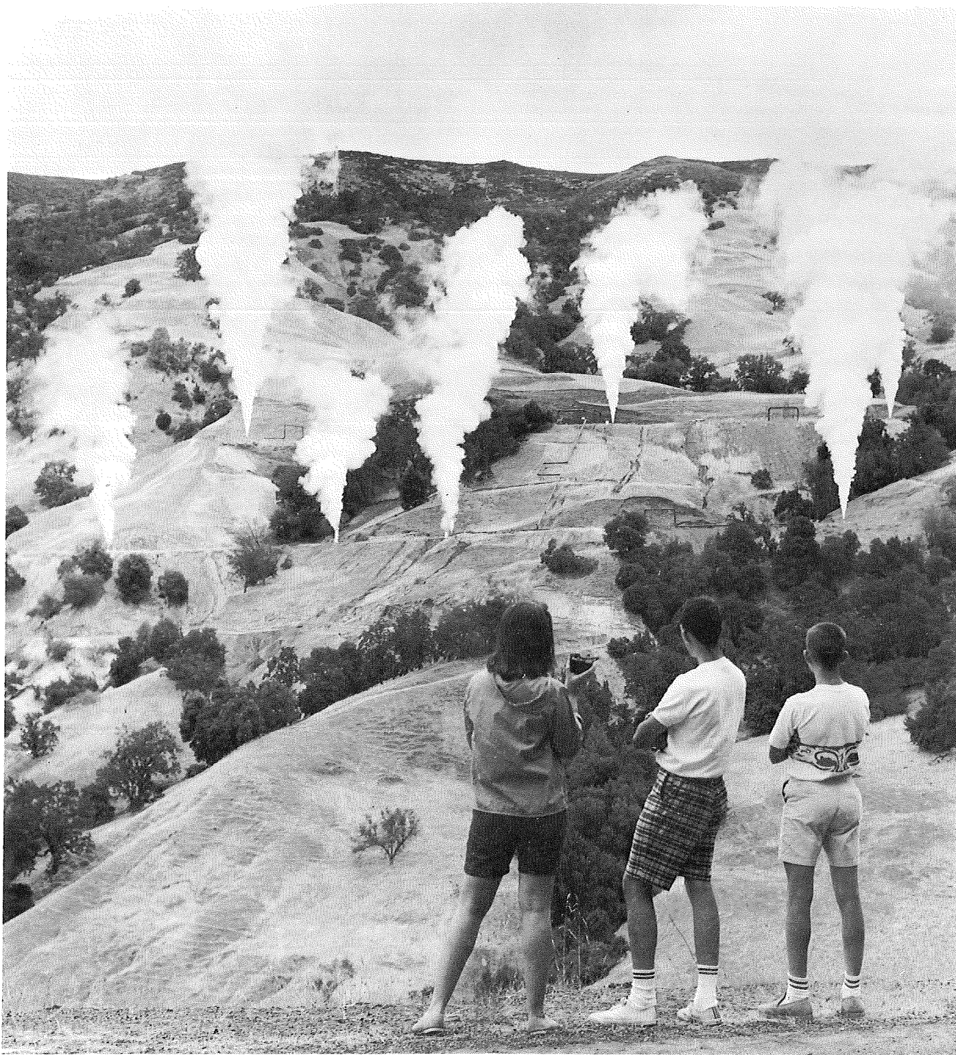
Photo No. 3. THOSE SMOKING HILLS--Tourists got a bonus display on the day of this big "blow out" at The Geysers. The eight wells in the Sulphur Bank area produce about 800,000 pounds of steam per hour. The blow out was conducted by Magma and Thermal Power Companies to remove accumulated subterranean debris prior to connecting five of the wells to piping which will carry 550,000 pounds of steam per hour to The Geysers Power Plant's generating Unit 3.
