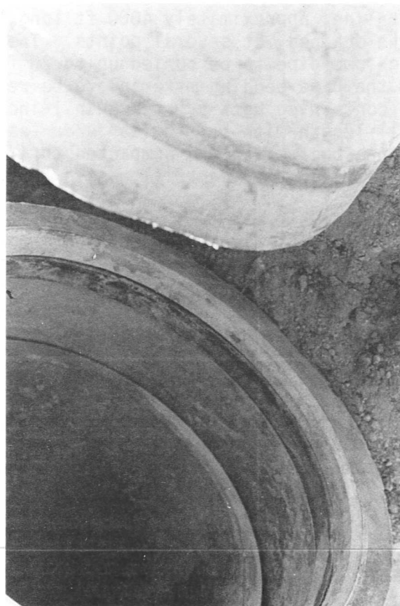
Fig. 2 View of coupling gasket between pipe sections
