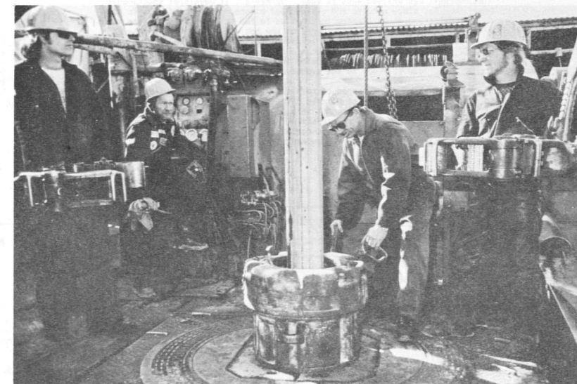
Drilling crew on the platform, near rotating table and drill rig controls
