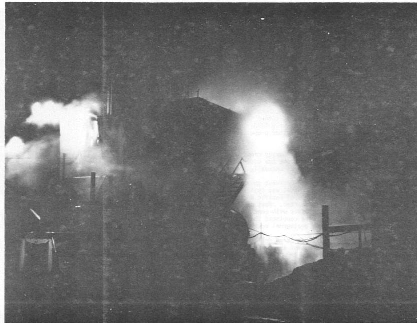
The nights of February 2, and 3, 1975, when the first well developed such a large flow of boiling water that the valves had to be closed and a plan developed for safely completing the well.
