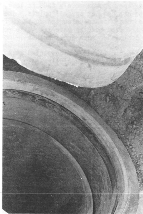
Fig. 2 View of coupling gasket between pipe sections
